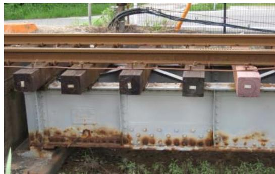
**Fig.1** Steel railway bridges with open deck system.
